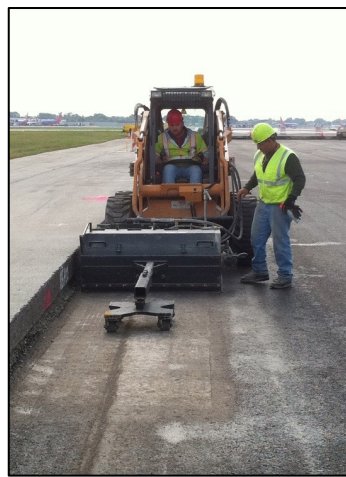
Ensuring accurate pavement depth at Chicago's Midway Airport
