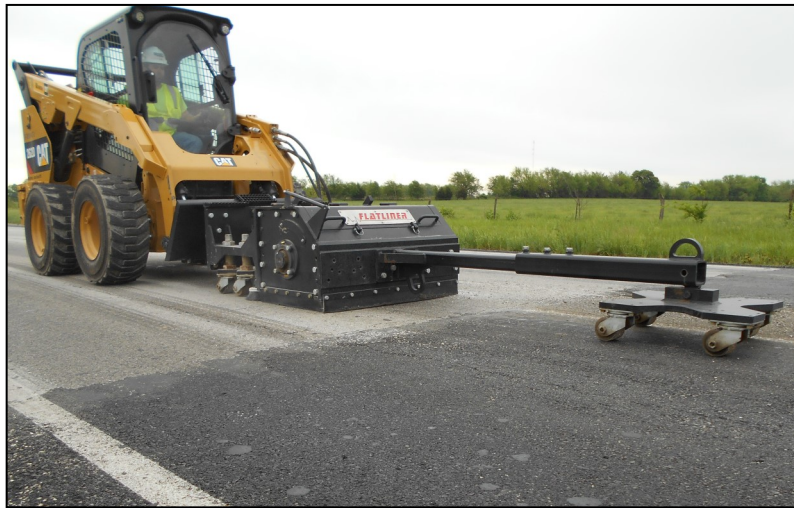
Corrective Grind—IRI Improvement
