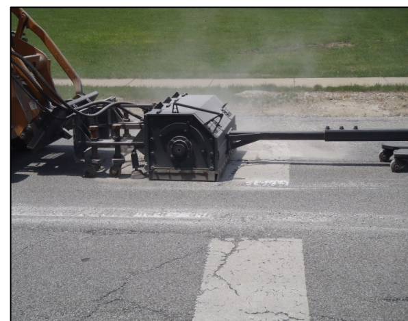
Pavement Markings and Coatings Removal
