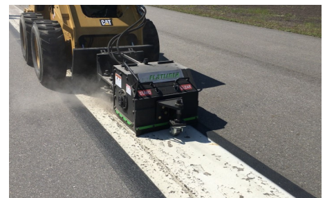
Airport Markings Removal with Flatliner FL24
