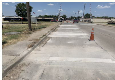
Concrete Joint Grinding with Edco Walk-Behind Grinder
