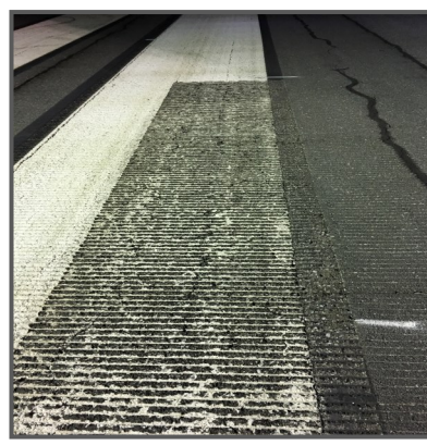
Runway Markings Removal with SS PCD Flat Bit
