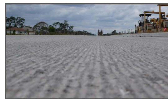
Micro Milled Surface with D-540 PCD
