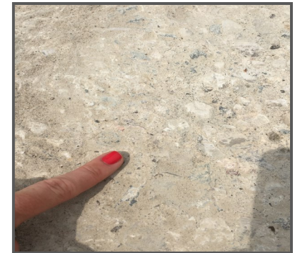
Concrete Texturing with SS PCD Flat
