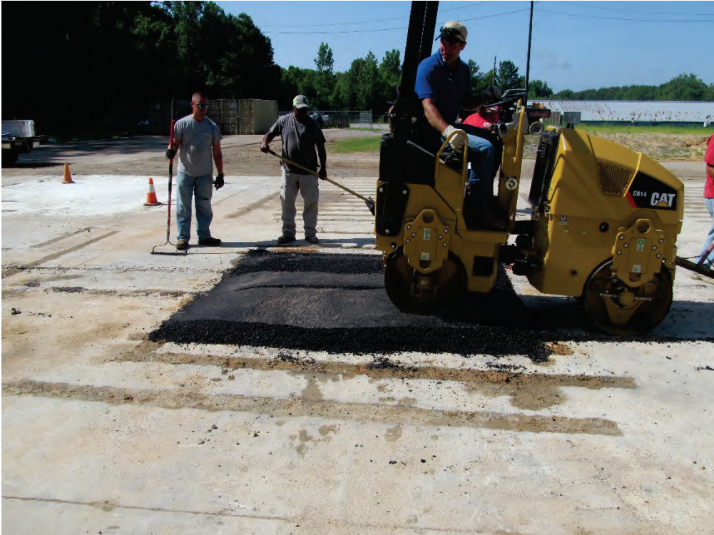
Figure 14. Compaction of AC using a small, tandem vibratory roller.
