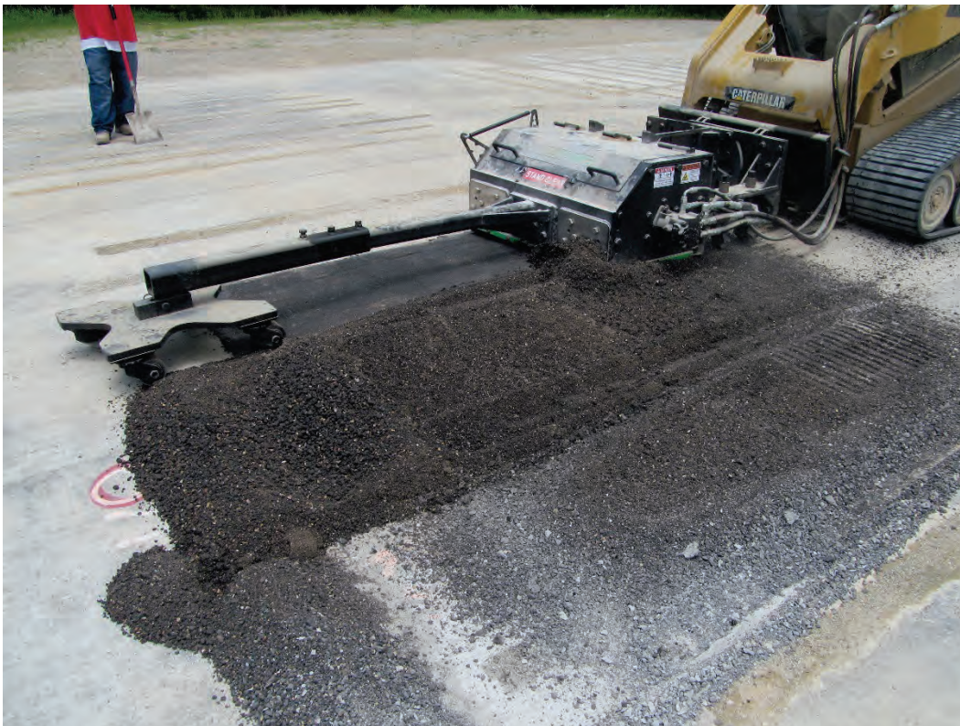
Figure 41. Planing 2-in.dome of crater Repair 6A with three equal passes.
