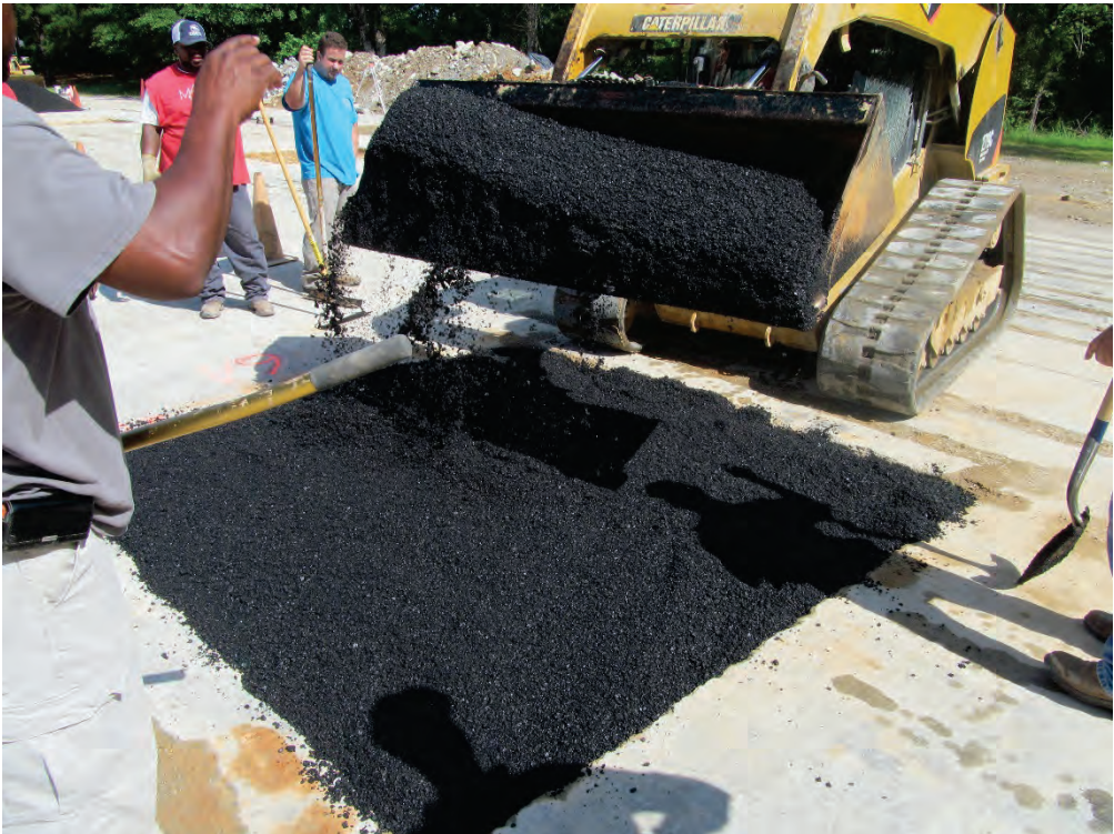
Figure 13. AC transported to crater repairs using skid steer.
