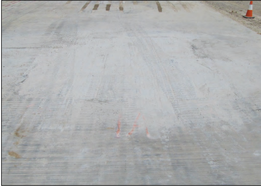
Figure 42. Repair 1A (RS) after multiple passes with the Flatliner.
