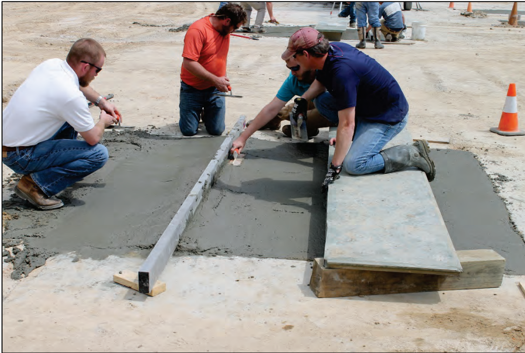
Figure 8. Forming PCC deficiencies using straight-edge beam.
