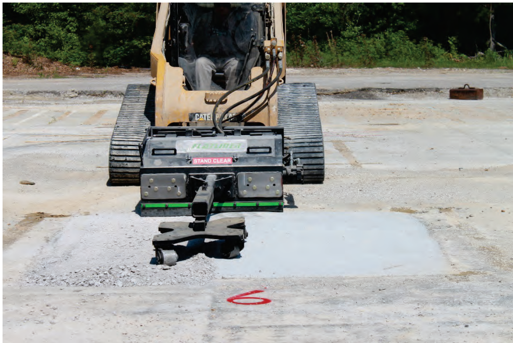
Figure 40. Planing 1.5-in.dome of crater Repair 6 with four equal passes.
