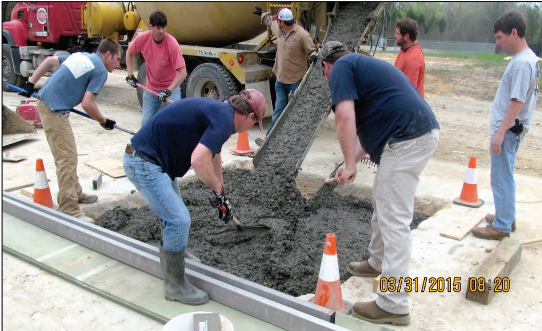
Figure 6. Placing PCC in Repair 1.
