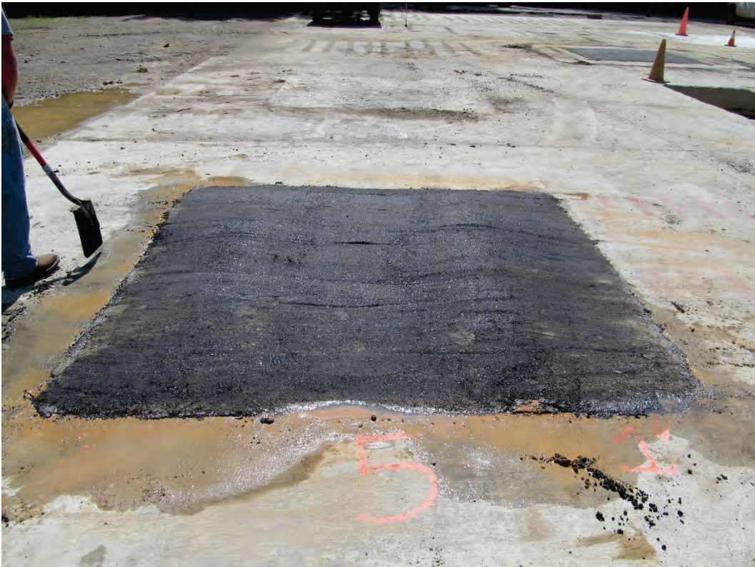
Figure 15. Completed AC crater repair.
