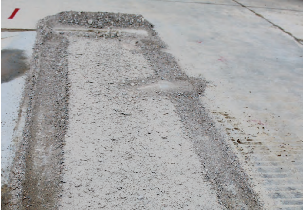
Figure 39. Surface of crater Repair 1 after one pass with Flatliner.
