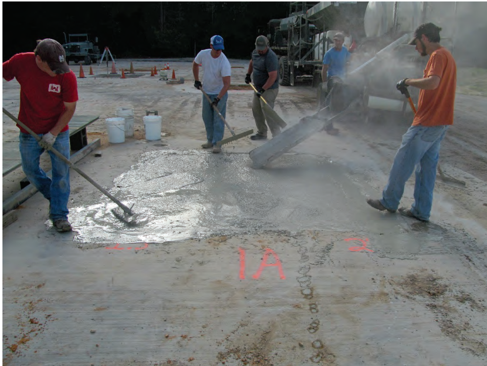
Figure 10. Placing RS concrete into crater Repair 1A.
