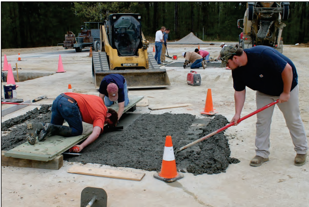
Figure 7. Using short scaffold to form center of repairs.
