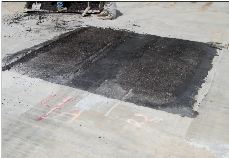
Figure 43. Repair 4A (AC) after multiple passes with the Flatliner.
