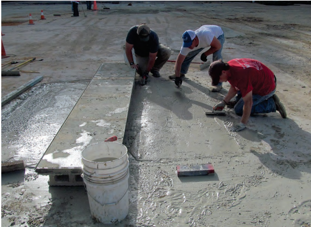
Figure 11. Forming RS concrete repairs to desired surface deficiencies.
