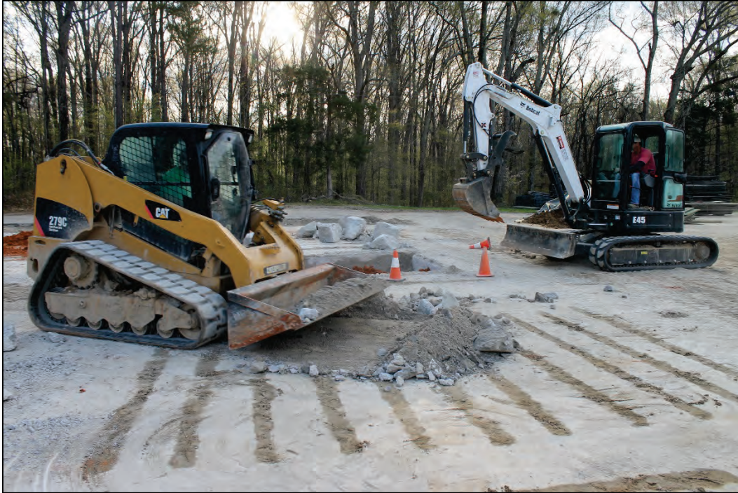
Figure 4. Removal of existing crater repairs and site cleanup.
