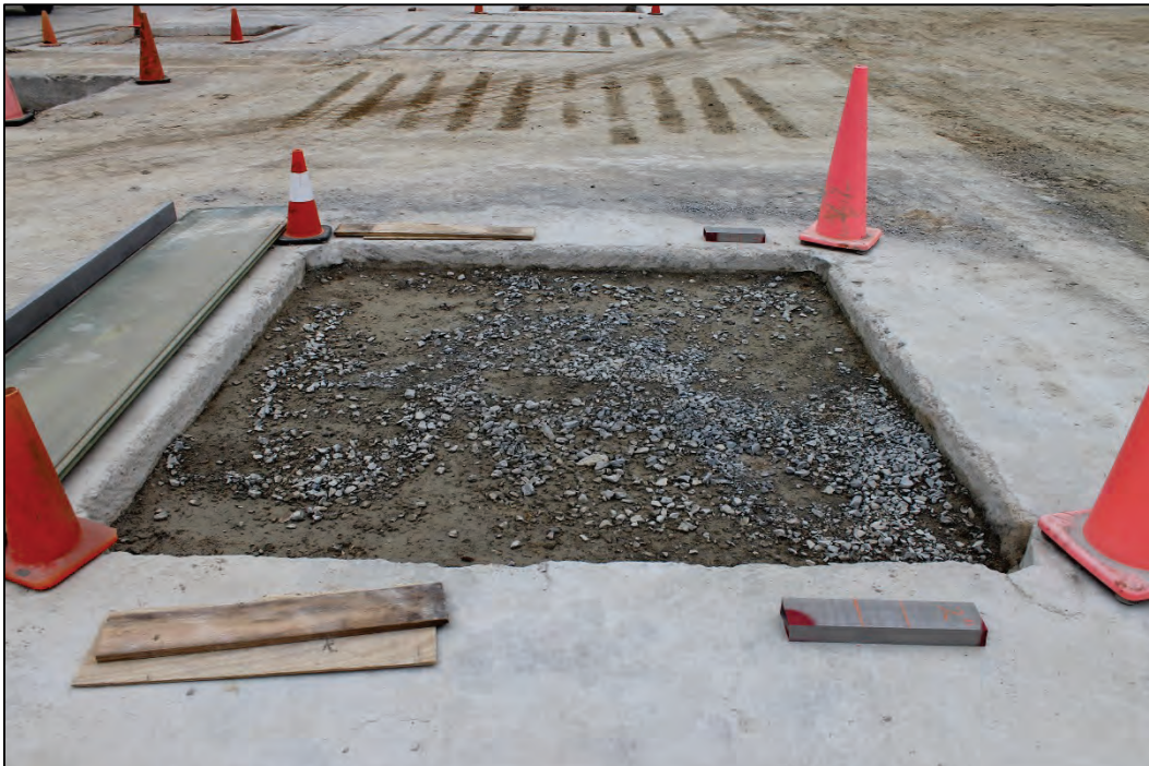
Figure 5. Completed breakout of existing crater.
