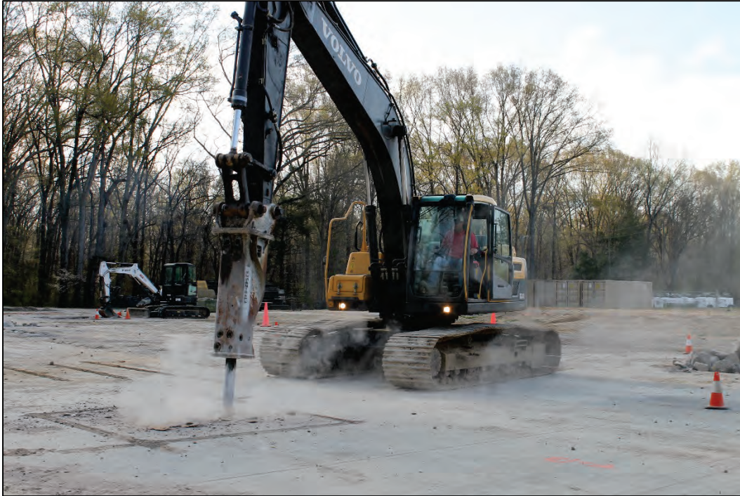
Figure 3. Breaking existing crater repairs with high impact jackhammer.
