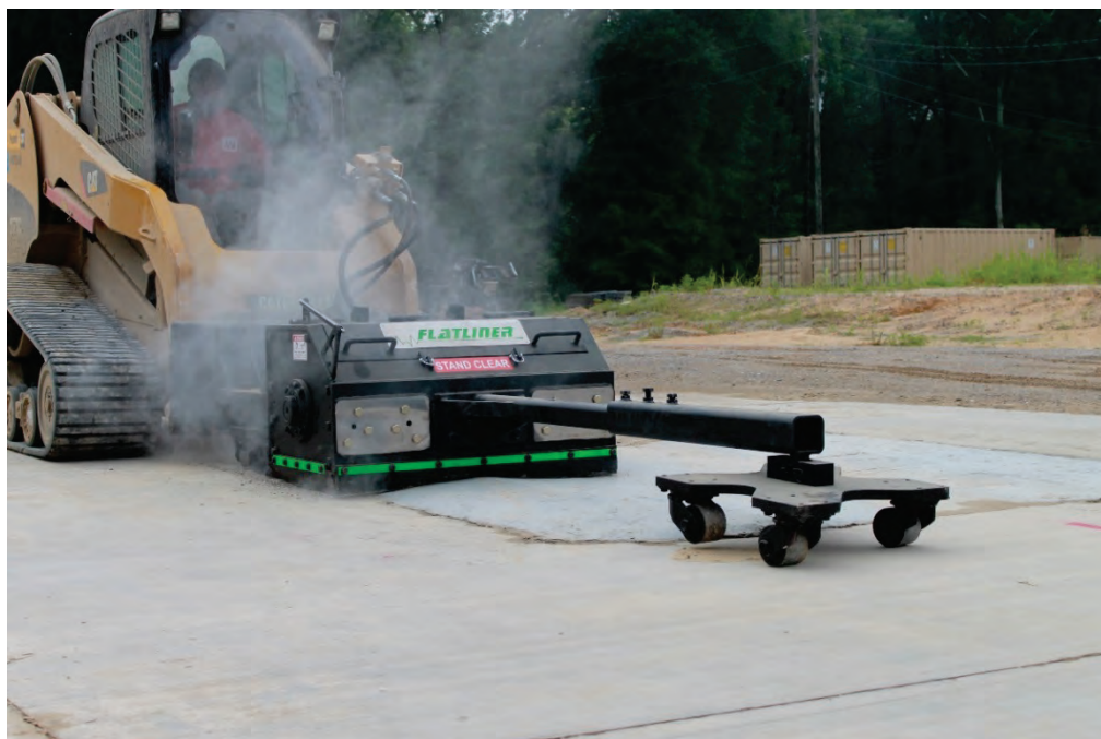
Figure 38. Planing 1.5-in. ridge of crater Repair 1 on north side of repair.
