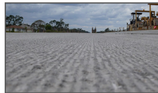
Micro Milled Surface with D-540 PCD
