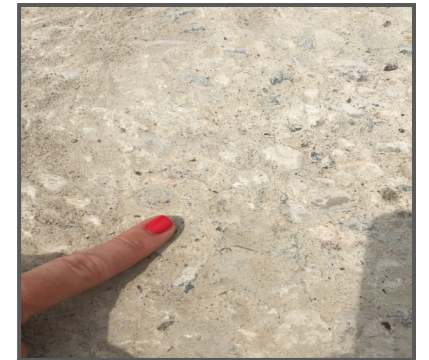
Concrete Texturing with SS PCD Flat
